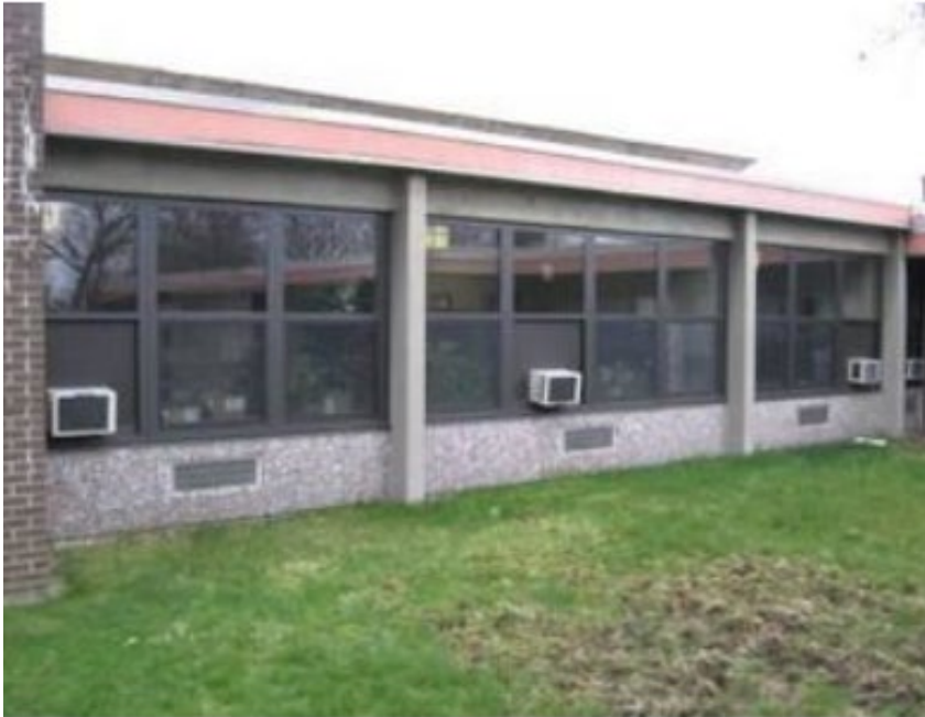
Insulated windows installed in 2003 and are in good condition
